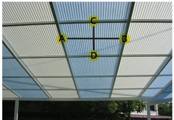
Spacing Recommendation (with 2 ribs side lapping) A to B : 950mm C to D : 750mm
